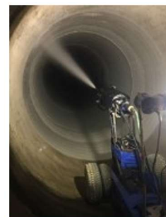
Robotic Installation Nukote Coating Systems
